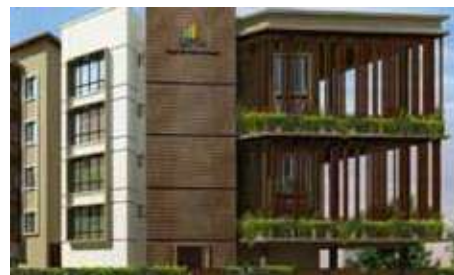
CASA CRESCENT Benson Town, Bangalore
