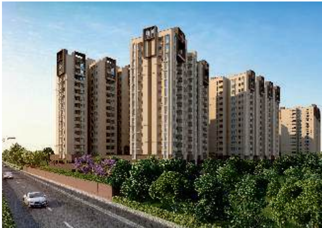
Sholinganallur, Off OMR
