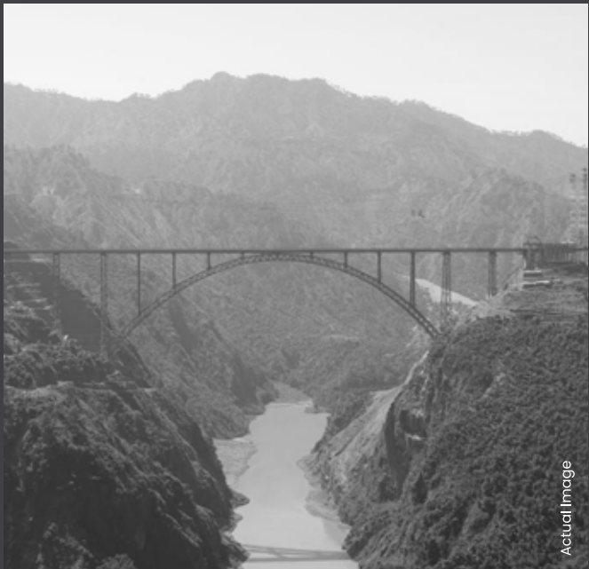
CHENAB BRIDGE, J&K
