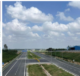
Bengaluru- Chennai Expressway
