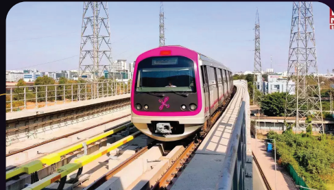
Bommasandra Metro Station
